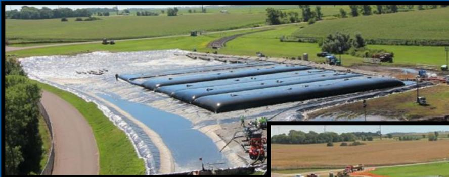
Dredged CCR materials were deposited in geotextile tubes on the dewatering pad - July 2016
